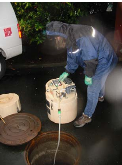
Environmental Service Technician, Terri Ayres, checks the automated sampler from a city waste stream.
